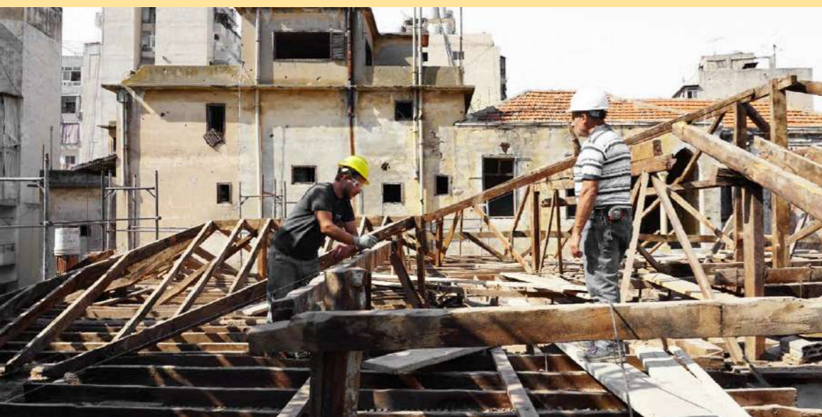
Photograph Trainee and carpenter assessing the condition of a wooden roof truss
